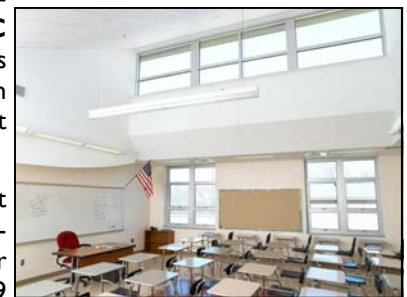
Top: Twenhofel Middle School in Independence, KY Bottom: Daylighting feature in classrooms allows for more natural light and reduces energy costs.
